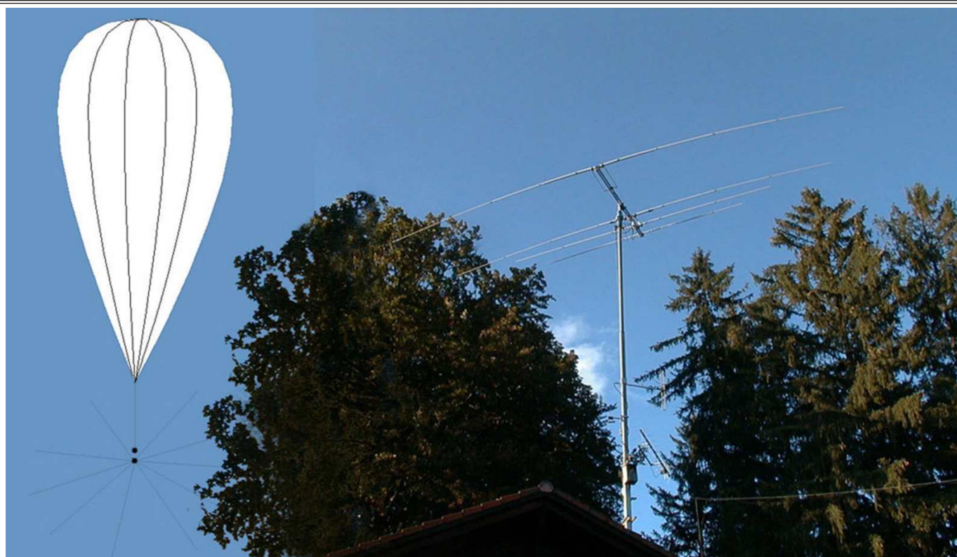
Cone Cage Vertical (1,8/3,5 MHz) h=20 meters d=8 meters. Yagi SOMMER XP40
